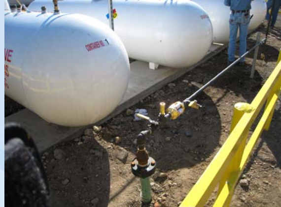
SIMAX 5 DRY TYPE FLASHBACK ARRESTOR INSTALLED. ELIMINATED HYDRAULIC FLUID STYLE
