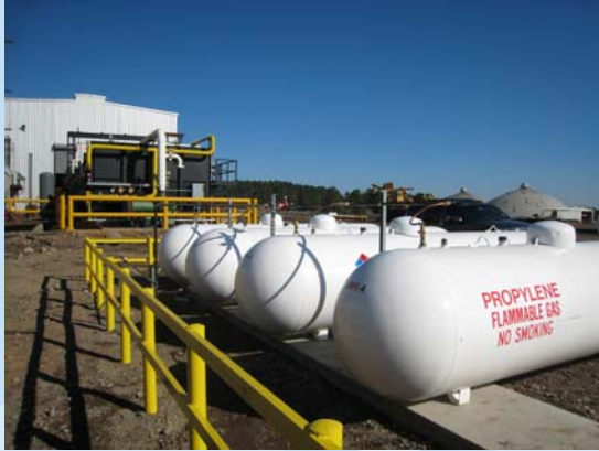
4-1,000 GALLON TANKS INSTALLED AND PIPED INTO PLANT
